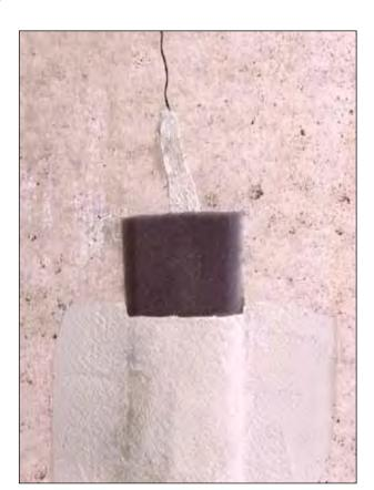
It's important to remember that the FlexiSpan® System is <u>not draining much water at all</u> since it incorporates a <u>seal</u> first! If it ever allows <u>any</u> water through the first seal, it would only be less than 5% of the original seepage. The drainage component is an innovative <u>second line of defense</u> to handle this minor seepage, if it ever occurs. This is what makes FlexiSpan® a special repair with completely predictable results:
