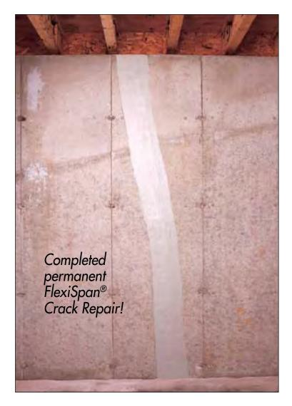
In some cases, your installer may elect to inject the crack with polyurethane resin or epoxy and to apply the FlexiSpan® System over the crack. Depending on the situation this may have advantages. It is usually unnecessary, as FlexiSpan® is a crack repair system on its own and is the most reliable method available.
