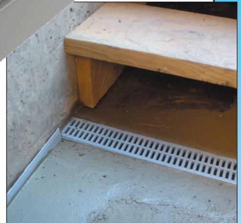
The design of the TrenchDrain allows for water to drain into the grate, flow into the patented WaterGuard sub-floor drainage system, and be pumped out of the home. TrenchDrain comes in several different styles: A large size used for traffic bearing and high flow conditions, and a smaller size
