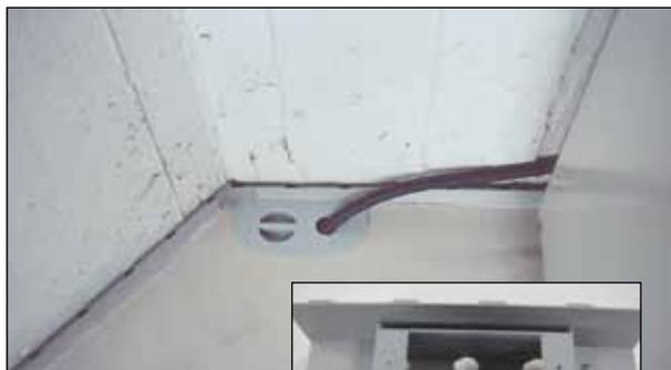
A WaterGuard® Port with removable cover is a nice feature. A knockout in the cover works well as a continuous dehumidifier drain outlet.
