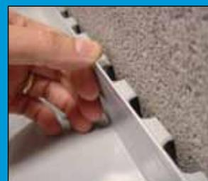
to drain any wall seepage, without allowing dirt and debris from the floor to enter. The **WaterGuard®** system is applicable to all types of foundations including block, poured concrete, stone, etc.
